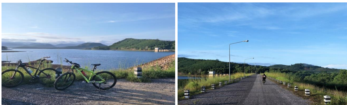
Figure 2 Khlong Sadao Dam
