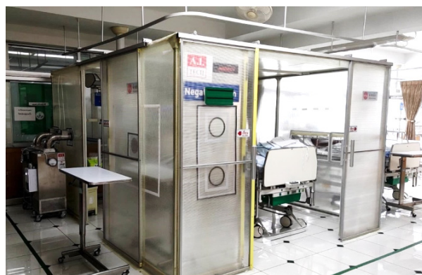
Figure 4 Negative pressure tent in neurosurgical intensive care unit
