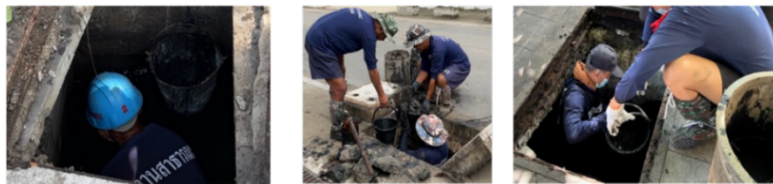
Task 3: Waste/Debris/Foreign Object Retrieval in the Sewer Pipe
