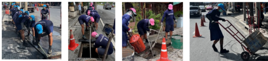
Task 4: Dragging the Cable Inside the Pipe (between access points 1 and 2)
