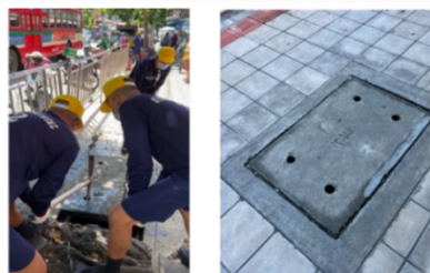
Task 6: Cleaning the Area and Closing the Drain Cover
