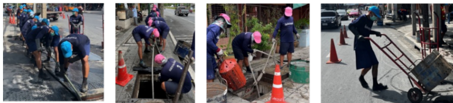
Task 4: Dragging the Cable Inside the Pipe (between access points 1 and 2)
