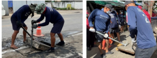
Task 2: Opening the Drain Cover
